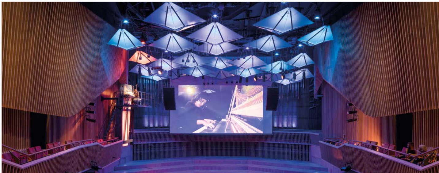
//Photo: Adam Mørk / Music School and Concert Hall Ventspils Windau – Lettland / Roller Screen System RUNWAY 10,0 x 7,5 m (32.8 x 24.6 ft)
