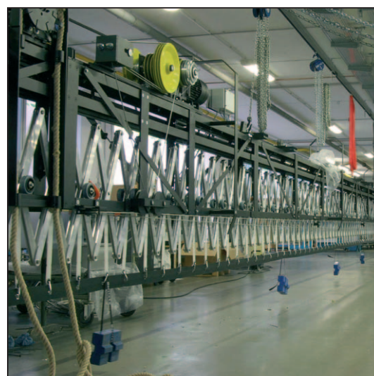
Congress Centre, Tashkent, Uzbekistan
